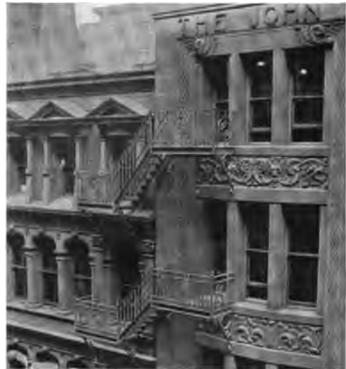
Fig. 2. Balcony around Fire Wall.
